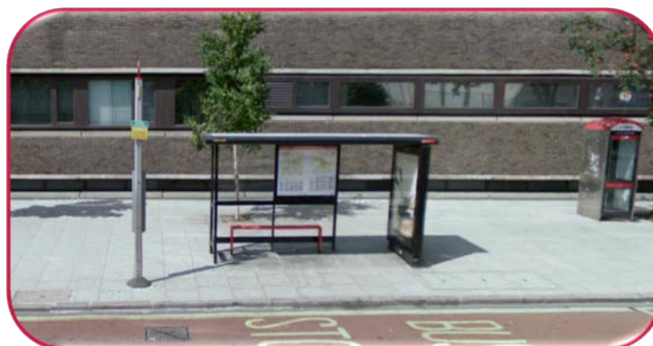
Figure 7.1: Goswell Road Bus Stop US
