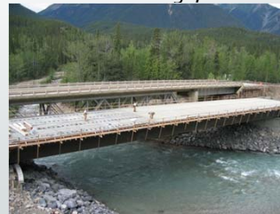
Trout River Bridge, Alcan Hwy.
