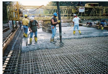
Mills Rd. Bridge, OH
